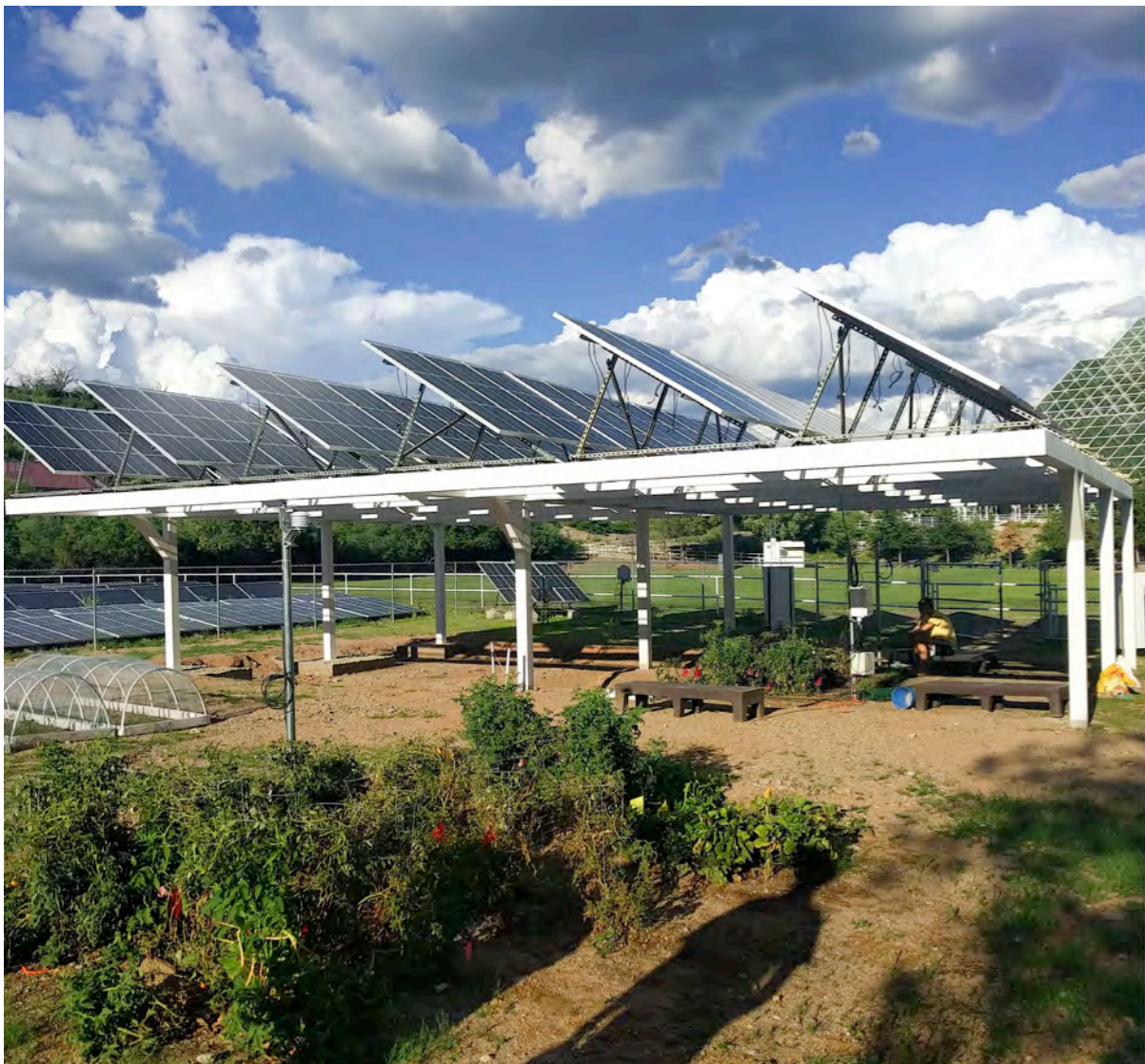
Figure 7. The co-location of agricultural under an elevated ‘overstory’ of PV panels has demonstrated increased production of some crop species (tomatoes, carrots, cabbages, chiltepin peppers, and kale) and increased water savings in the irrigation needed for additional spring and summer crops including red and yellow chards, purple, tepary, and cow beans, cilantro, and Japanese eggplant.
